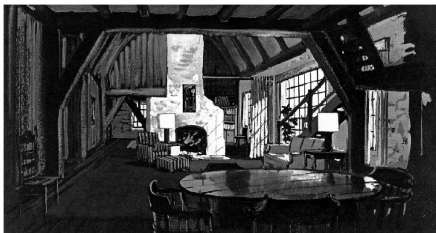
Figure 6.5 Drawing of the Old Mill after renovation.
