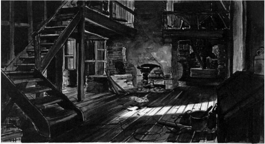
Figure 6.3 Drawing of the Old Mill before renovation.
